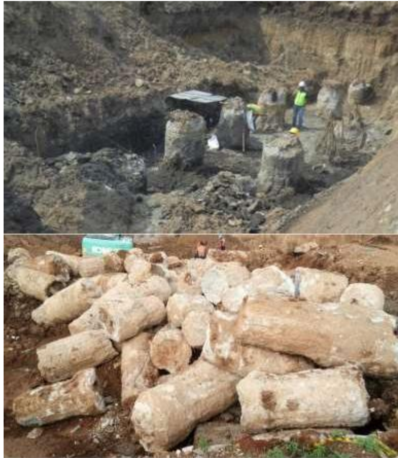
Gambar 4.22 Pondasi Bore Pile
